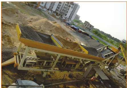
In Line Storage Bins
