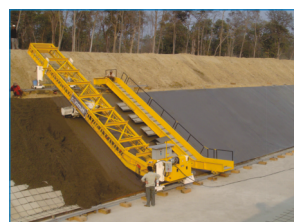
Concrete Canal Paver
