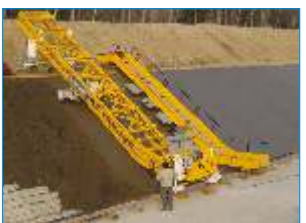
Concrete Canal Paver
