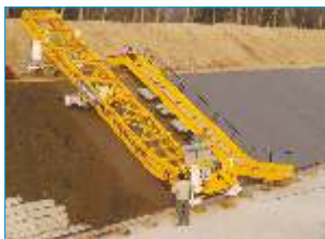
Concrete Canal Paver
