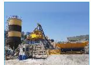
Tora Batching Plant
