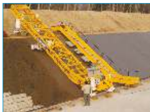
Concrete Canal Paver
